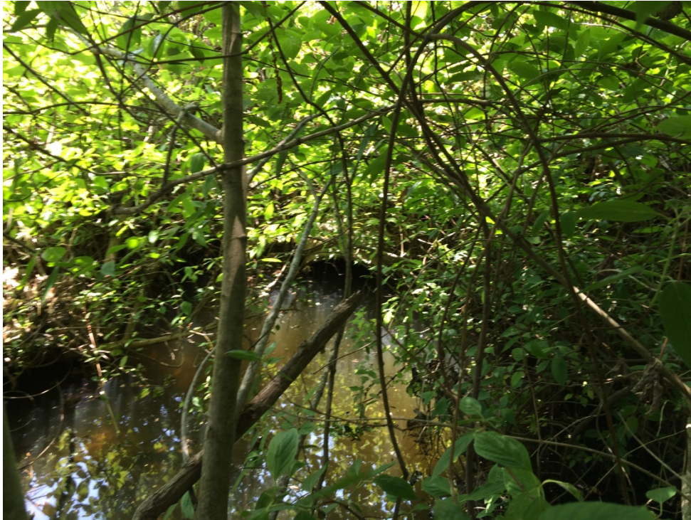
Photo 26 Outfall 86 – broken pipe under Church Street (NCDOT owned)
