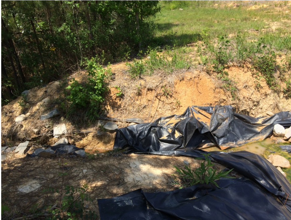
Photo 25 Outfall 85 – downstream of outfall
