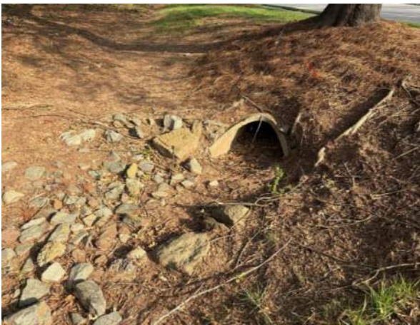
Representative photo of a culvert on the Subject Property.
