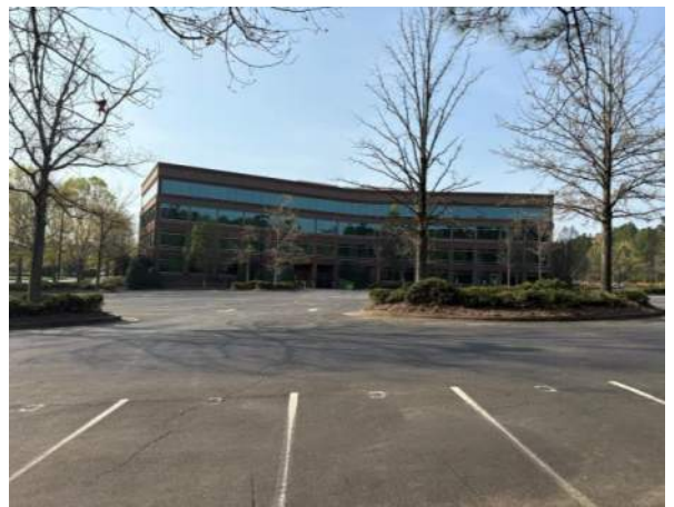
Representative photo of an adjacent office building and parking lot.
