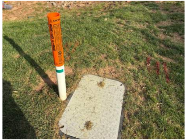
Representative photo of the fiber optic cable along Paramount Parkway.
