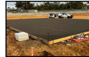
Photo 1 – Example of pitch square constructed and ready for turf installation before outfield subgrade preparation has been completed.
