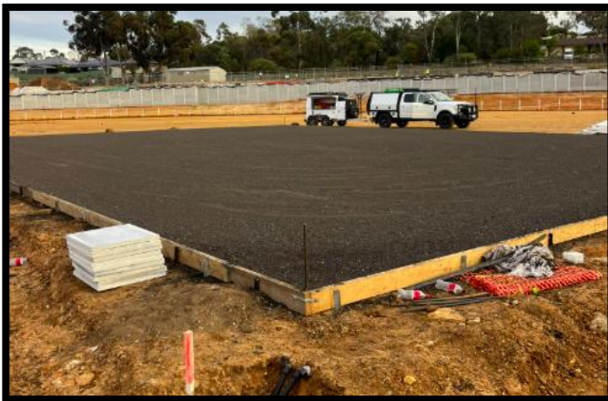
Photo 1 – Example of pitch square constructed and ready for turf installation before outfield subgrade preparation has been completed.
