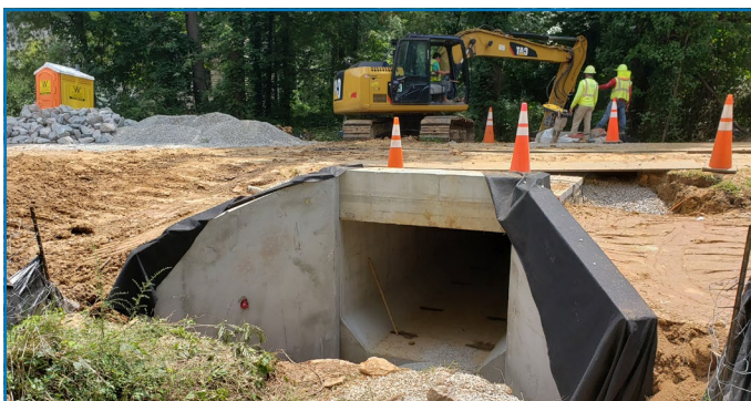
Green-Fairview Flood Reduction Construction
