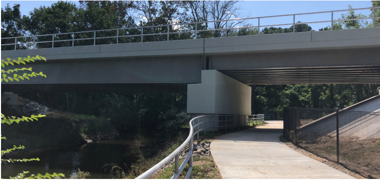
Crabtree Creek Greenway NC Railroad Underpass
